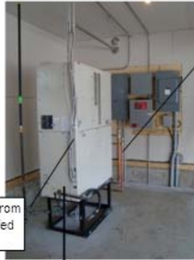
Water pipes, to and from house, supply all space and domestic hot water heat.
