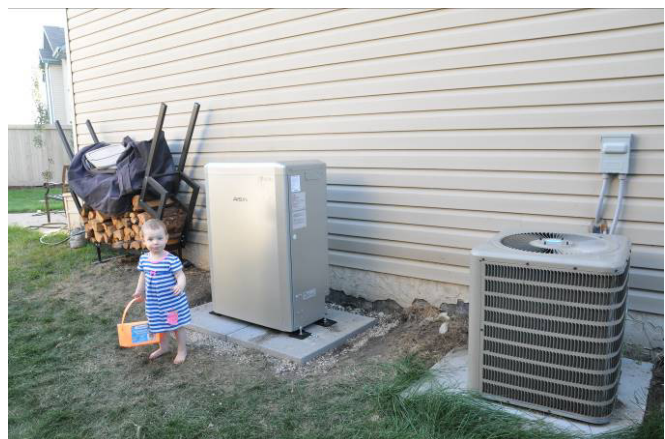
mCHP unit outside home
