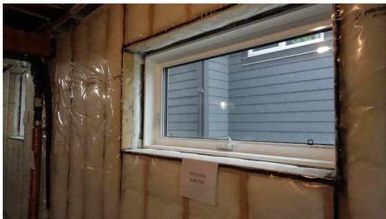
6. Double stud walls and triple pane windows in the basement
