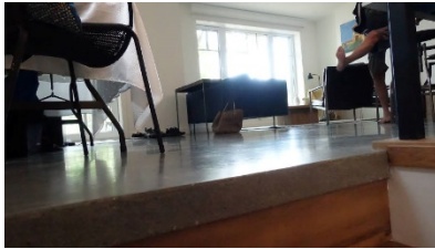
4. A concrete floor and south facing windows for passive solar gain.
