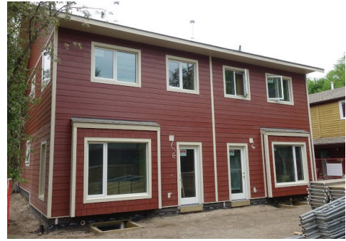
9. A town home wrapped with new exterior insulated panels.
