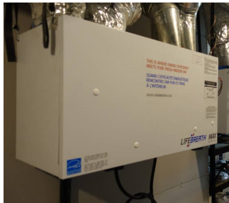
8. A heat recovery ventilator (HRV).
