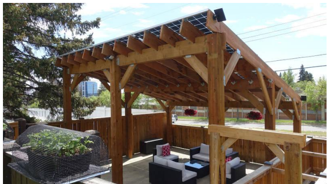
1. A solar pergola with translucent solar modules.
