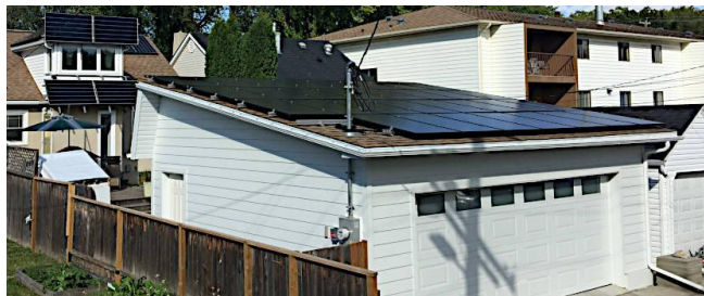
10. This 1949 home has R14 walls but still gets to net-zero with geothermal heating and a large solar array on the custom garage.
